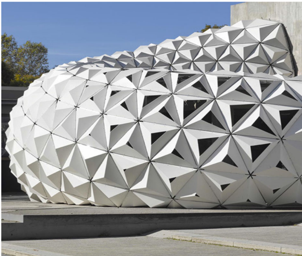
Fig. 3 Spiky modules of the ArboSkin Pavilion in Stuttgart (Germany) made of bioplastic containing over 90% renewable materials (freely downloaded from the Institute of Building Structures and Structural Design of the University of Stuttgart)
